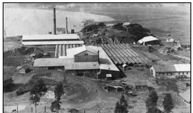
Hoffman Kilns near McNear Brickyard c. 1904
